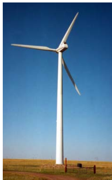
Figure 6-2: Horizontal axis wind turbine (Source: NREL, US DOE)
