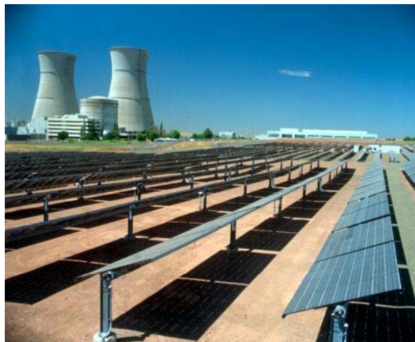
Figure 5-1: Field of fixed, tilted PV arrays in the exclusion zone around a nuclear power station, California (Source: NREL, DOE)
