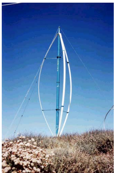
Figure 6-1: Vertical axis wind turbine (Source: NREL, US DOE)
