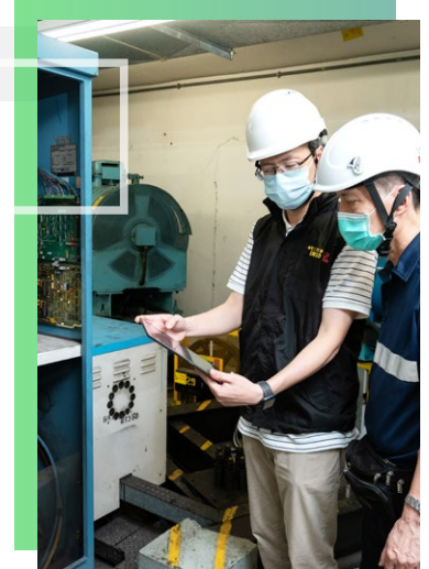
Safe access to plant items, which require frequent and regular maintenance, shall be provided
