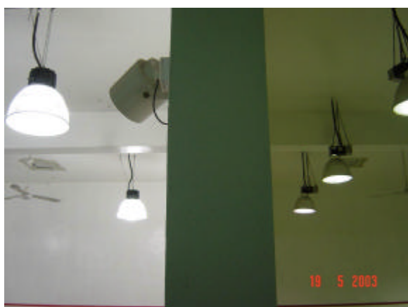
Figure 15 - Direct illuminance comparison between court 2 (induction) and court 3 (HID)
