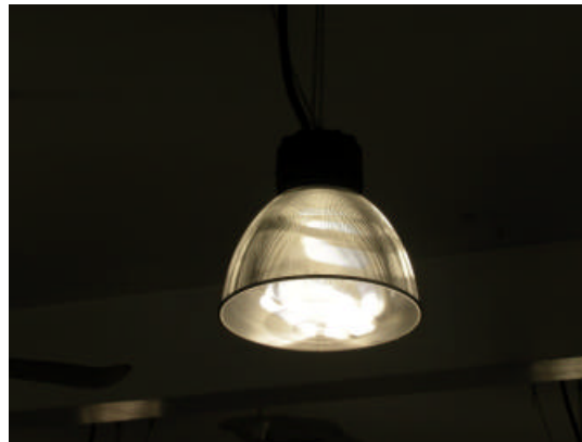
Fig. 10: New high-bay luminaire with 2x150W external-coil induction lamps
