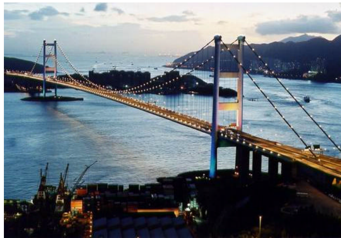
Fig. 4: Induction lamps used on ropes and bridge sides in Tsing Ma Bridge
