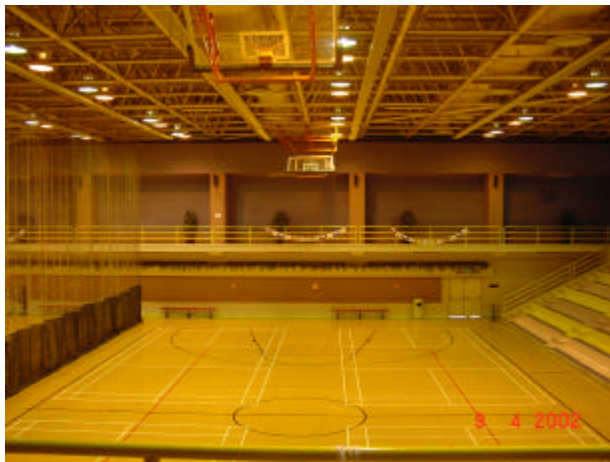
Fig. 9: Existing lighting environment with HID lamps in Kowloon Bay Indoor Games Hall
