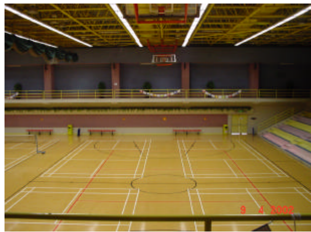
Fig.10: New lighting environment of the High Output T5 Lighting in Kowloon Bay Indoor Games Hall
