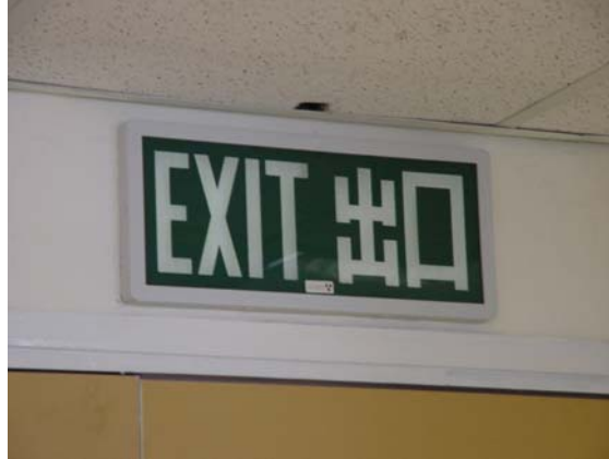
Fig. 3: New self-luminous EXIT sign installed at EEO
