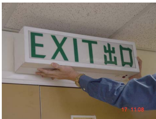
Fig. 1: Conventional EXIT sign using 18W T8 fluorescent lamp & power pack
