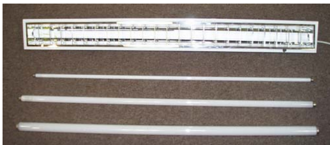
Fig. 7 Physical Size of T5 Luminaire under tested as compared with T8 & T12
