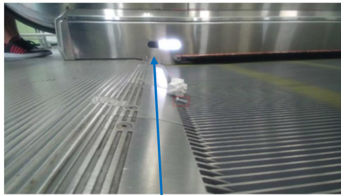
Video Camera for Escalator Comb Object Identification System
