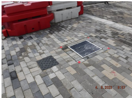
Pair of manholes accommodating GNSS equipment (Manhole with solar panel cover encloses GNSS receiver and battery, remaining manhole houses GNSS antenna)
