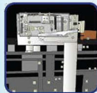
4. Install an advanced car door mechanical lock and door safety edge
