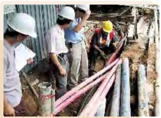
工地附近如有地下電纜,施工前必須採取合理措施。 Reasonable safety measures must be taken prior to works in the vicinity of underground electricity cables.
