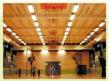
A high-output T5 lighting systems is now in operation at East Kai Tak Indoor Games Hall (see photo above). Preliminary results indicate an energy saving of over 40 per cent when compared with the existing high bay lighting system using High Intensity Discharge lamps (see photo on left).
