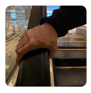
When pulled by hand, the handrail has <u>no</u> slackening
