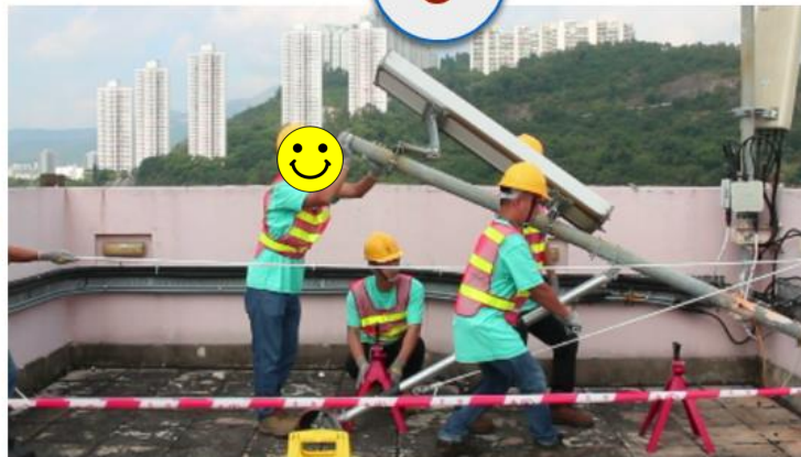
• Reverse the operation after the work
