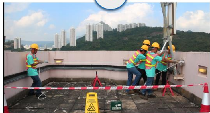
• Erect & secure the pole safely
