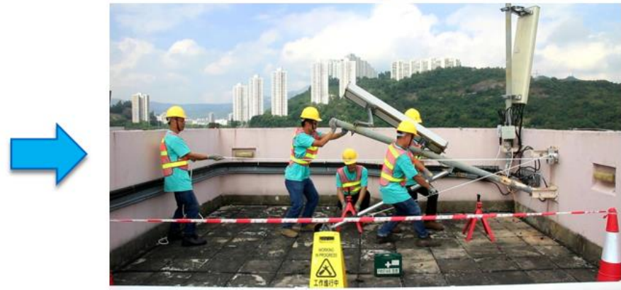
• Lower the Antenna Pole using the Loader
