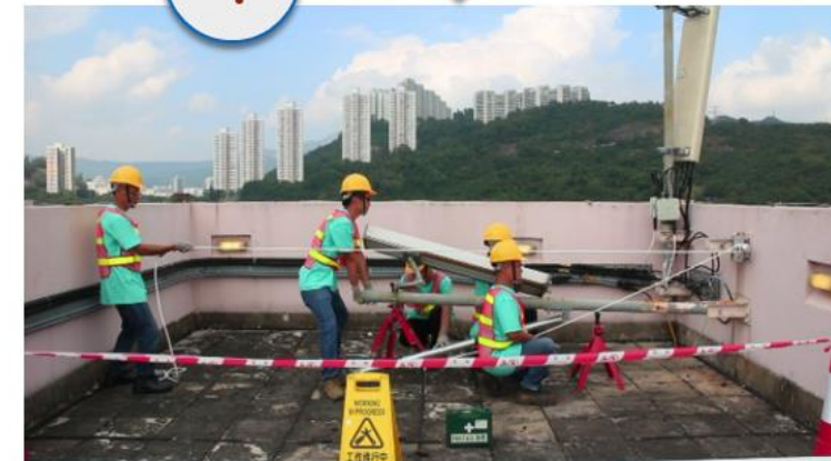
• Perform work required on ground safely
