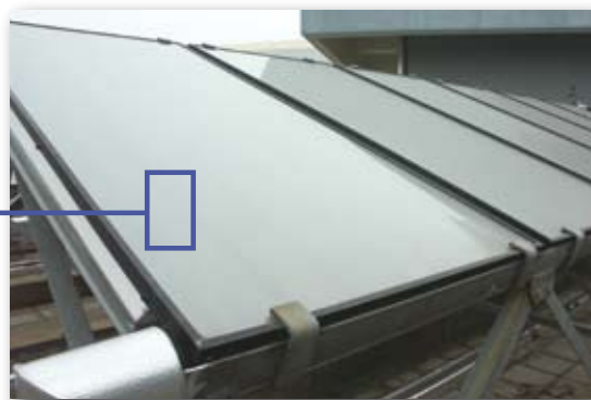
Appearance of Flat Plate Type Solar Thermal Collector 平板型太陽能集熱器外貌
