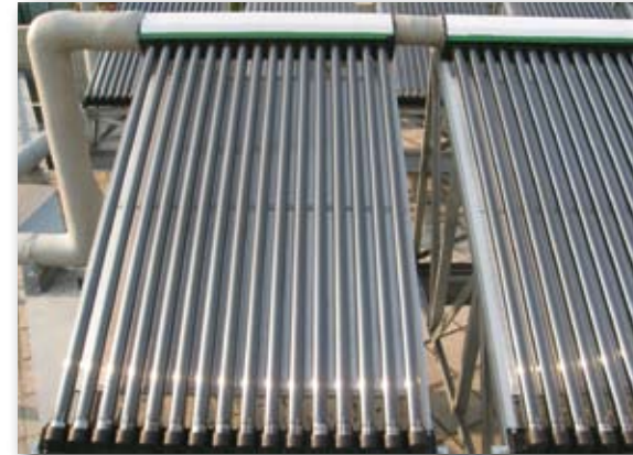
Fig. 3a - Evacuated Jacket Solar Thermal Collector
