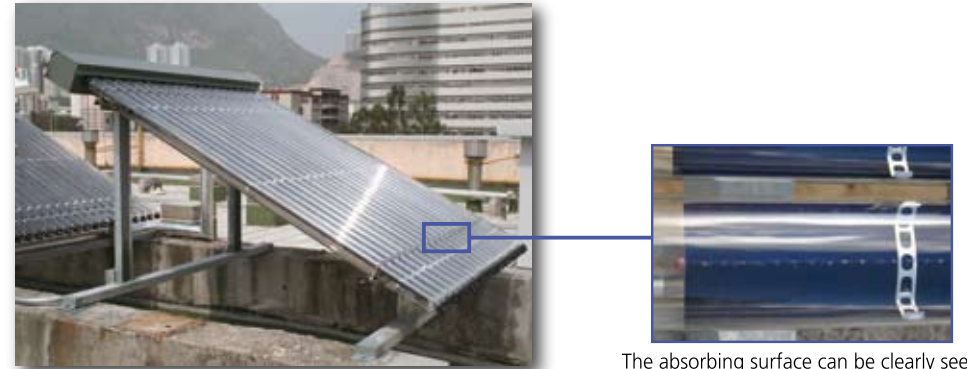
Appearance of Evacuated Heat Pipe Solar Thermal Collector 熱管式真空管太陽能集熱器外貌
