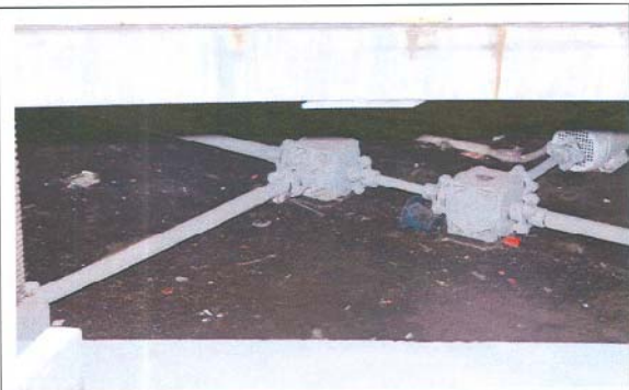
Fig. 13: Water within the range underneath the movable platform in Ngong Ping Terminal
