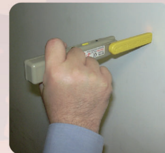
▲ 使用金屬探測器確定牆內喉管位置 Use metal detector to detect the exact position of concealed pipes and conduits.
