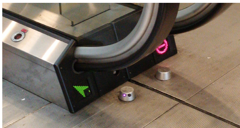
Figure 8.5.7 (b): Example of floor mounted sensors
