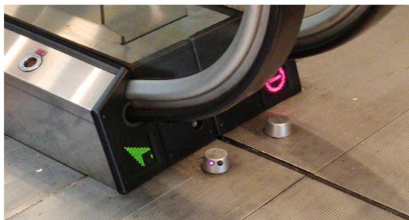
Figure 8.5.7 (b): Example of floor mounted sensors
