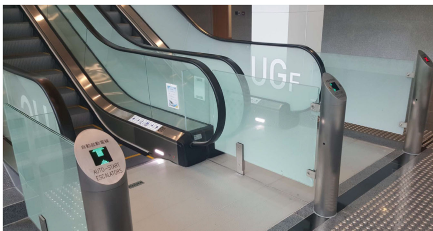
Figure 8.5.7 (a): Example of pole mounted sensors
