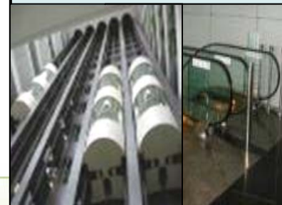
Lift and Escalator Installation
