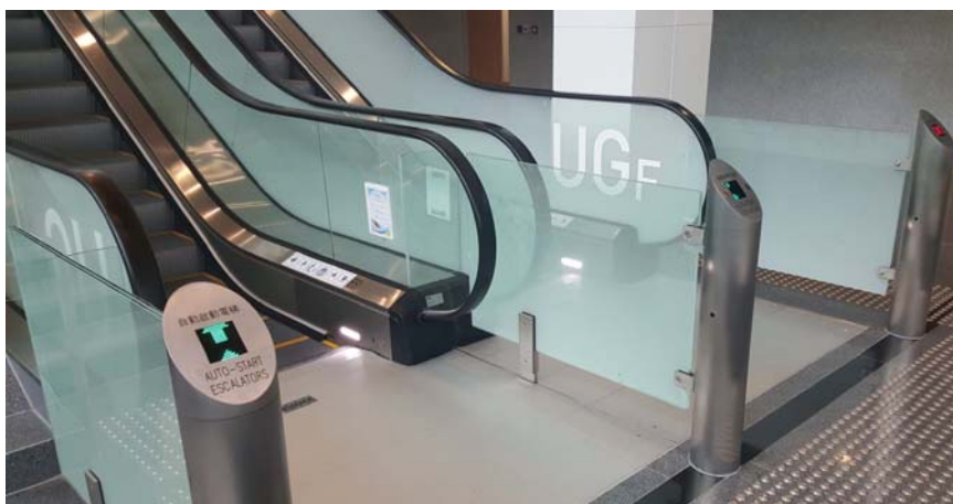
Figure 8.5.7 (a): Example of pole mounted sensors
