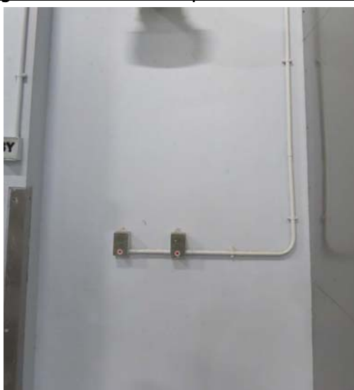
Figure 6.10.7 (a): Example of CO/NO Sensor
