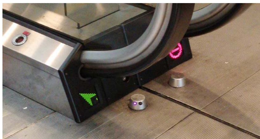
Figure 8.5.7 (b): Example of floor mounted sensors
