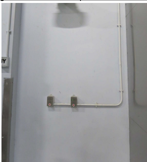
Figure 6.10.7 (a): Example of CO/NO Sensor
