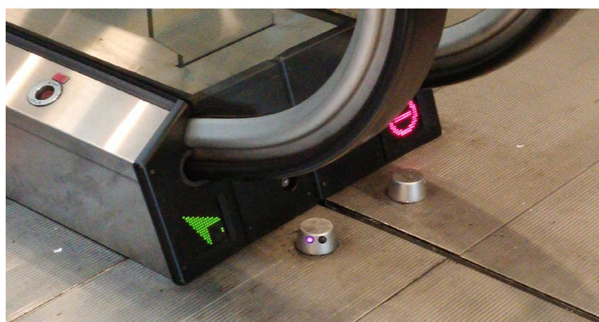
Figure 8.5.7 (b): Example of floor mounted sensors
