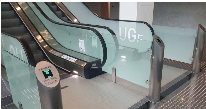
Figure 8.5.7 (a): Example of pole mounted sensors
