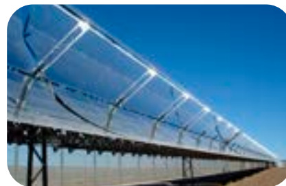
Parabolic Troughs at Andasol in Spain
