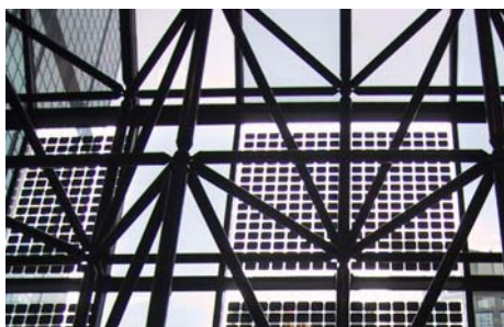
Fig. 7. Skylight Sub-system – Interior view
