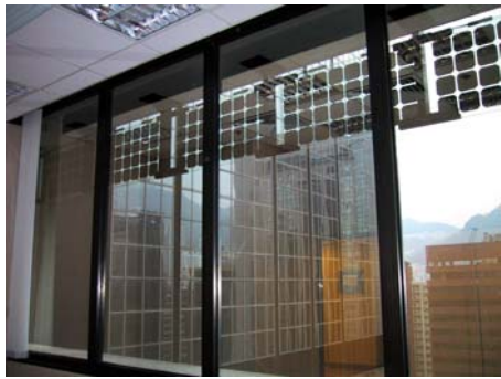
Fig. 6. Sun-shade Sub-system – Interior View
