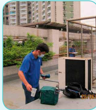
檢查冷卻塔 Inspection of cooling tower
