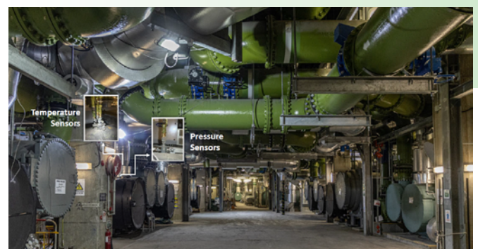
■ 收集運作數據的傳感器 Sensors that collect operation data
