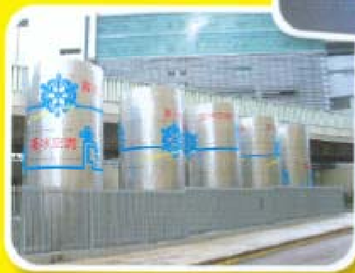
Slurry Ice Storage Tanks
