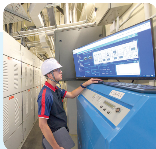
我們在海關總部大樓安裝了新設備，包括傳媒接待室的大屏幕和先進混音器（左），以便更精確調校聲音；此外，還有智能電掣房監察系統（右），以加強電力裝置的維修保養。 We installed new equipment in the Customs Headquarters Building, including a large monitor and an advanced audio mixer at its media briefing room (left) for more precise control of sound, as well as a smart switch room monitoring system (right) to strengthen maintenance of electrical installations.
