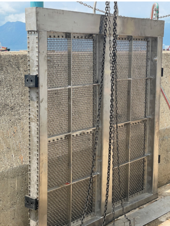
由機電署研發的智能防污海水濾網，利用超聲波技術及設有智能污垢指數分析功能，可清潔海水濾網和防止生物膜在濾網上形成。該項目在第三屆亞洲創新發明展覽會—香港上獲得金獎。圖為時任機電工程署署長彭耀雄先生(左五)與獲獎團隊。Developed by the EMSD, the Smart Antifouling Seawater Screen adopts the ultrasound technology and has a smart fouling index analysis function for cleaning seawater screens and averting the formation of biofilm on them. The project won a gold medal at the 3rd Asia Exhibition of Innovations and Inventions Hong Kong. Pictured are Mr Pang Yiu-hung, the then Director of Electrical and Mechanical Services (5th left), and the winning team.
