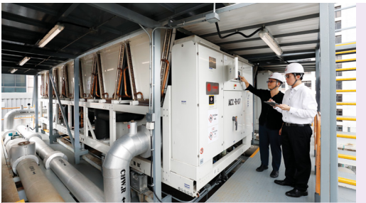
機電署把瑪嘉烈醫院的氣冷式製冷機組，更換為採用低全球升溫潛能值雪種的機組，有效減少溫室氣體排放。鑑於該款雪種具輕度易燃特性，項目團隊加裝了雪種監察系統，以確保運作安全。 The EMSD has replaced the air-cooled chillers at Princess Margaret Hospital with units using a low-GWP refrigerant, effectively reducing greenhouse gas emissions. Given the mild flammability characteristics of the refrigerant, a refrigerant monitoring system has been installed to ensure operational safety.
