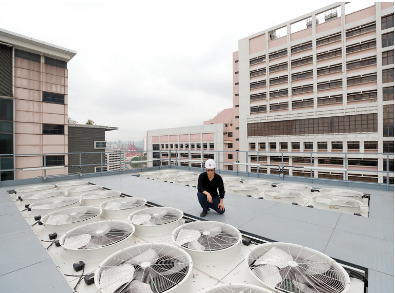
機電署把瑪嘉烈醫院的氣冷式製冷機組，更換為採用低全球升溫潛能值雪種的機組，有效減少溫室氣體排放。鑑於該款雪種具輕度易燃特性，項目團隊加裝了雪種監察系統，以確保運作安全。 The EMSD has replaced the air-cooled chillers at Princess Margaret Hospital with units using a low-GWP refrigerant, effectively reducing greenhouse gas emissions. Given the mild flammability characteristics of the refrigerant, a refrigerant monitoring system has been installed to ensure operational safety.
