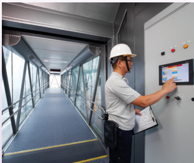
在新啟德郵輪碼頭，我們的工作人員透過船橋內的控制屏測試及校驗登船橋的操作。 At the new Kai Tak Cruise Terminal, our staff conducts testing and commissioning of the Seaport Passenger Boarding Bridge operation through a control console inside the Bridge.
