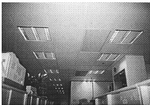
Fig. 10 Lighting after retrofit with new T5 luminaires
