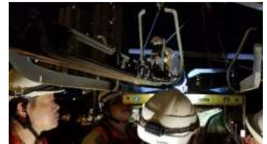
Detect signs of arcing and high temperature on section insulator
