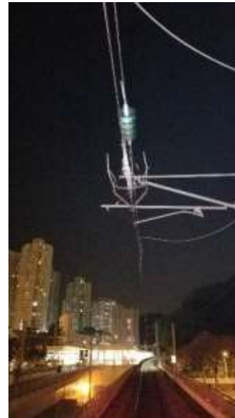
Detect signs of arcing and high temperature on section insulator
