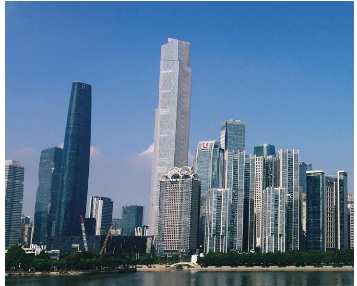
The tallest building in the image above is the Guangzhou Chow Tai Fook Finance Centre
