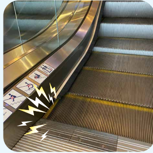
There is no abnormal sound when the escalator is operating
