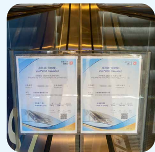
A valid use permit and the emergency contact number of the registered escalator contractor are displayed in a conspicuous position
