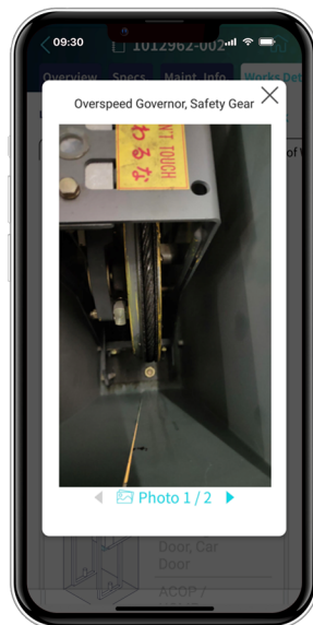
Figure 4 – Photo of lift maintenance works
