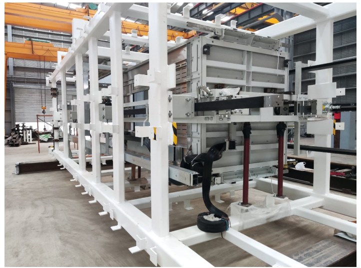
A lift car pre-installed in the lift shaft structure
