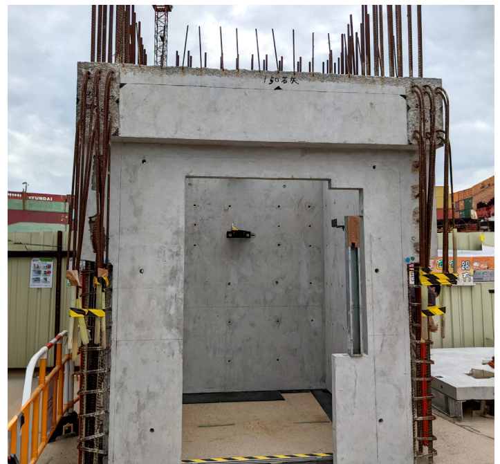
An MiC Lift Shaft
