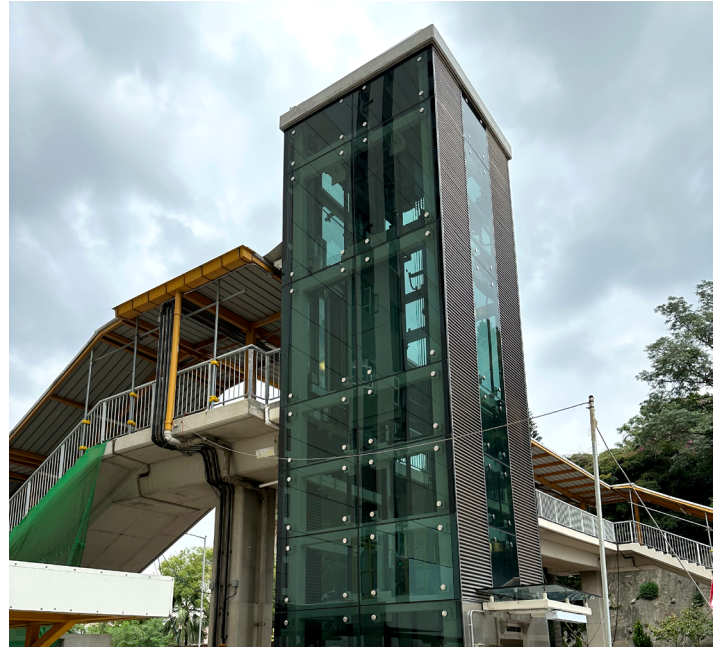
A MiC lift at a footbridge
