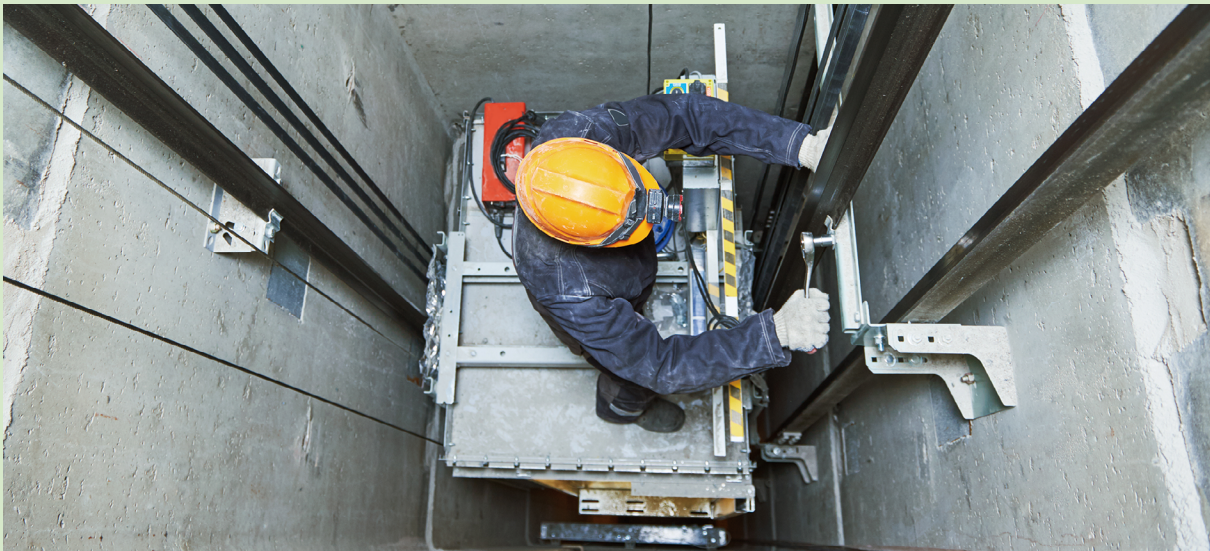
A worker working in the lift shaft
