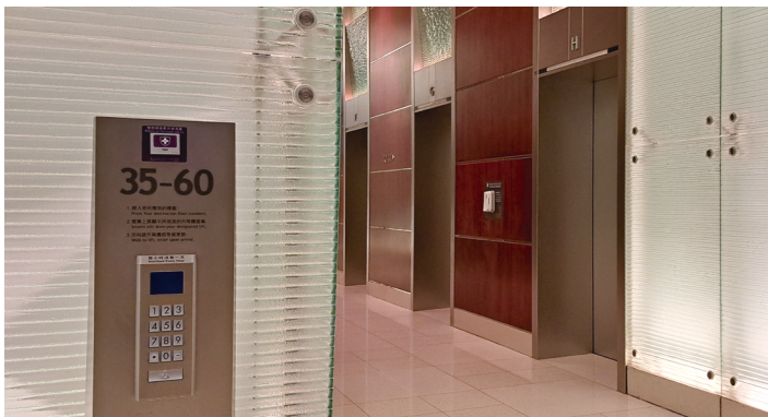
A building equipped with DCS
