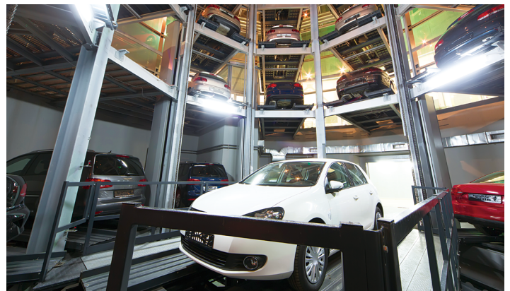
Circular shaft lifting system
