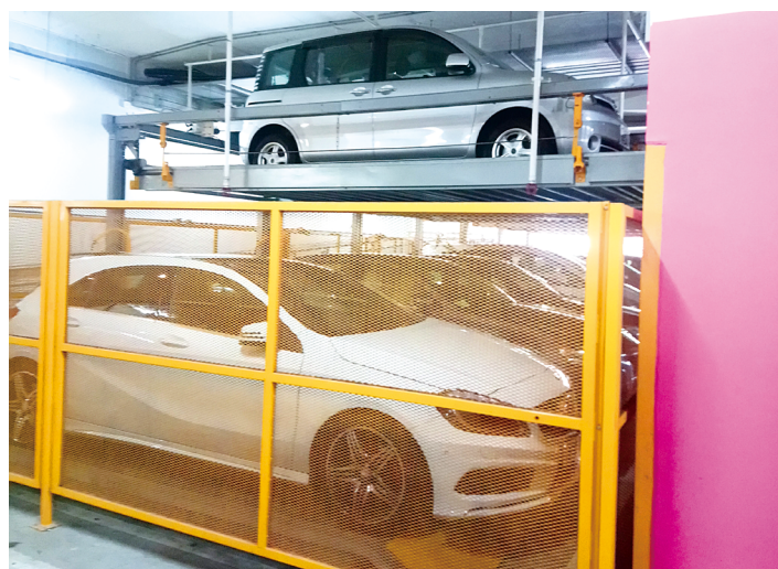
After installing the puzzle stacking system, the space behind the columns can also be used for parking
