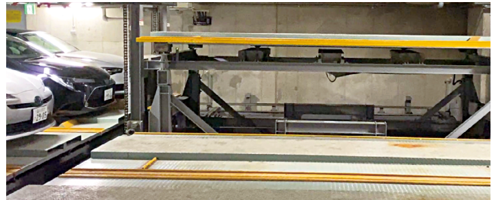
A horizontal circulation system equipped with a lifting platform
