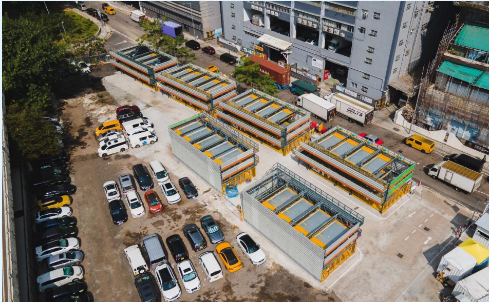
Overview of the car park at Hoi Shing Road, Tsuen Wan
