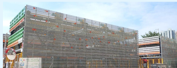
An MVPS with windshields installed
