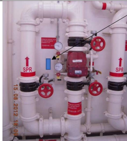
RFID Tag for control valve set
