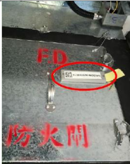
RFID Tag for fire dampers
