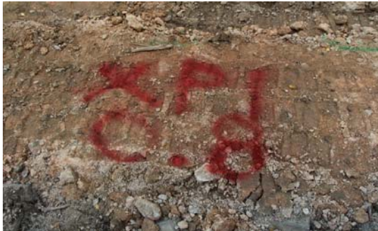
Photo 5 (Marked the cable alignment & depth on site)
