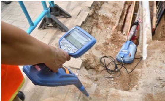
Photo 5 (Marked the cable alignment & depth on site)
