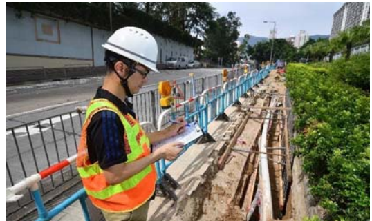
Photo 6 (recorded Marked the cable alignment & depth)
