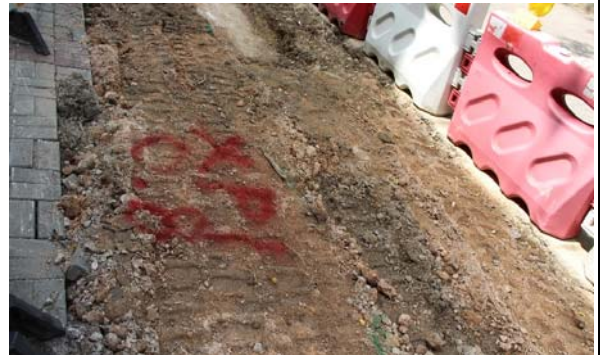
Photo 4 (Marked the cable alignment & depth on site)
