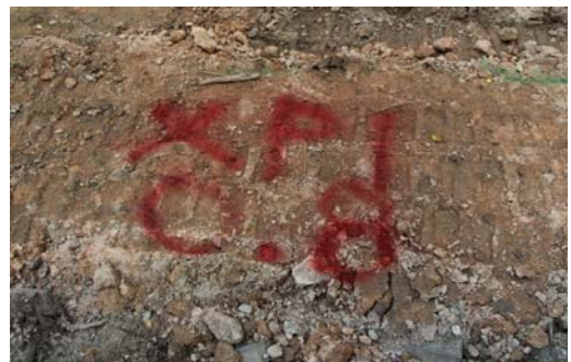
Photo 4 Marked the cable alignment
