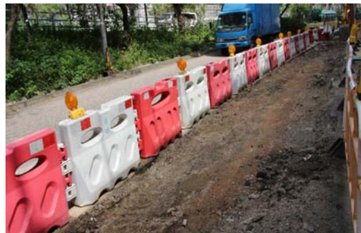
Photo 4 Marked the cable alignment
