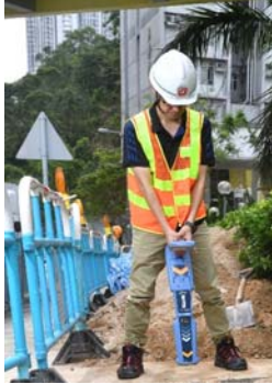
Photo 3 Marked the cable alignment
