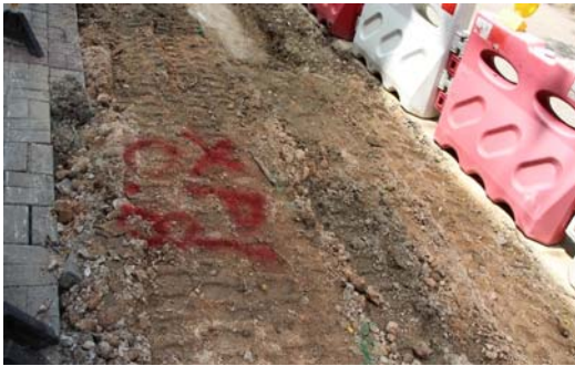
Photo 3 Marked the cable alignment
