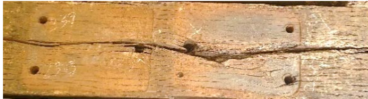
Figure 19 : Rotten timber sleeper
