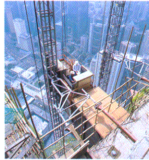
Builders' lifts are among the various mechanical installations under EMSD's regulation
