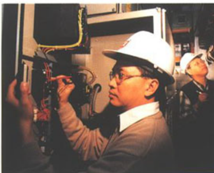
Safety inspection of communal electrical installations in private buildings
