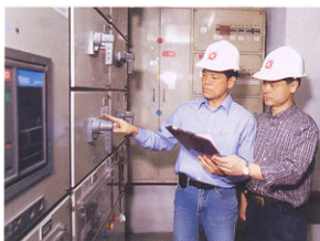
EMSD conducts about 9,000 site inspections on electrical installations each year
