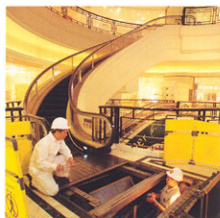
Inspectors inspecting an escalator in a shopping mall in Causeway Bay
