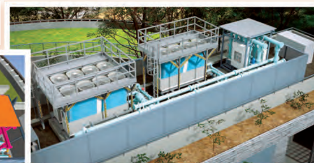
大龍獸醫化驗所製冷機組 The chiller plant of Tai Lung Veterinary Laboratory
