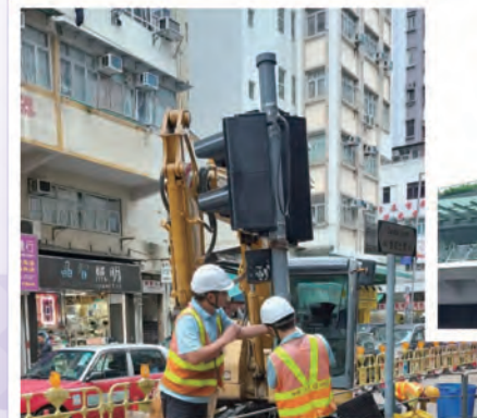
緊急修復受惡劣天氣破壞的交通燈。 Emergency repair to the traffic lights damaged in adverse weather.
