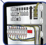
6. Install an obstruction switch to protect the suspension ropes
