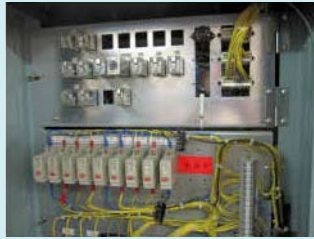
Obstruction switch installed in the control panel
