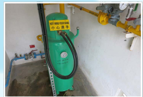
▲ Figure 2: A change-over device
