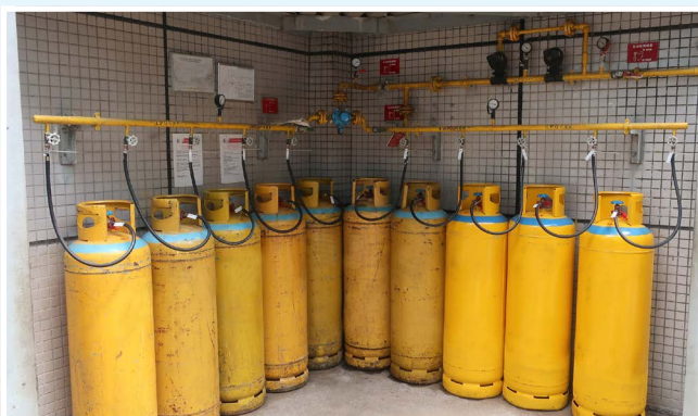
▲ Figure 1: An LPG cylinder store
