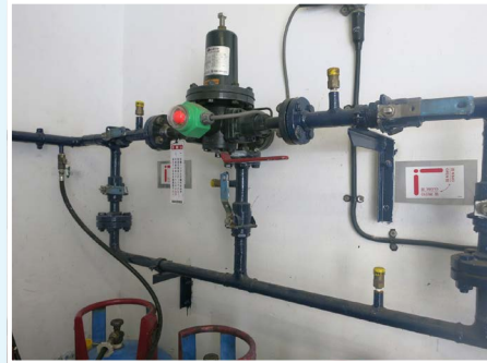
▲ Figure 2: A change-over device
