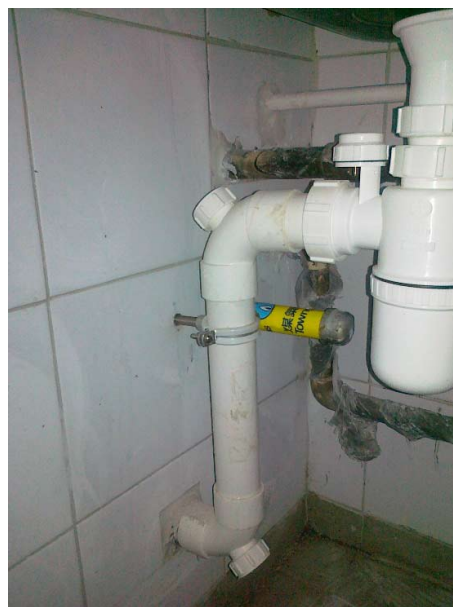
▲ Photo1: Marking of a live gas pipe in a unit in which the town gas supply has been disconnected
