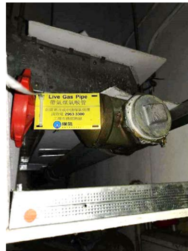
▲ Photo 2: Marking of a live gas pipe with town gas supply
